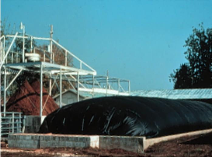
*An operational anaerobic digester*
